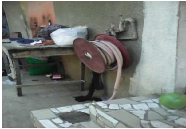
Figure 1. Non-functioning Fire Hose Reel in the Central Part of the Formal Section of Garki Model Market (Source: Researcher's Field Work, 2017)
